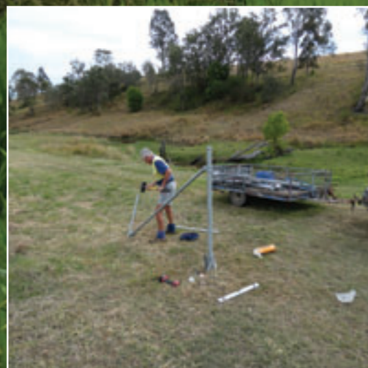
Insert left: Dave Gillespie installing Gallagher Mega Anchor around the chain of ponds site Insert right: New electric fencing up around the chain of ponds site Background: The chain of ponds site now protected by Gallagher fencing
