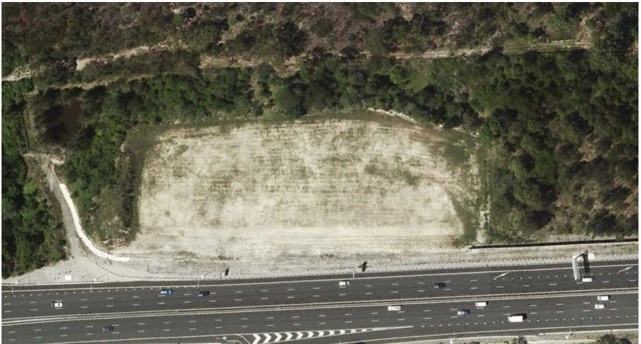
This picture shows the cleared area of site on the Northern side of the M2 Motorway which is between Khartoum Rd to the East and Christie Rd to the West.
